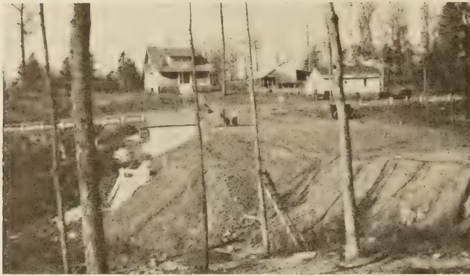
Clay fill at 10-foot level
